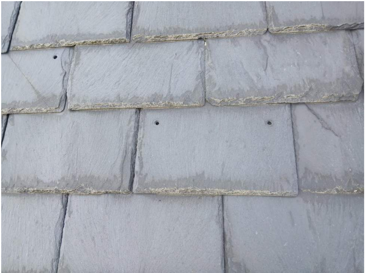
Image 1 - Incorrectly installed slate shingle example
