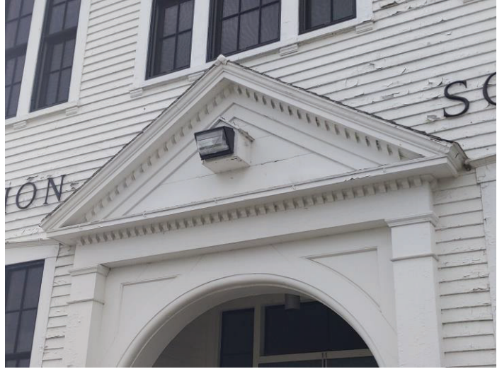
Image 4: 20 th century paint schemes often whitewashed historic trim and siding. Fortunately, much of the wood detailing is still in good shape.
