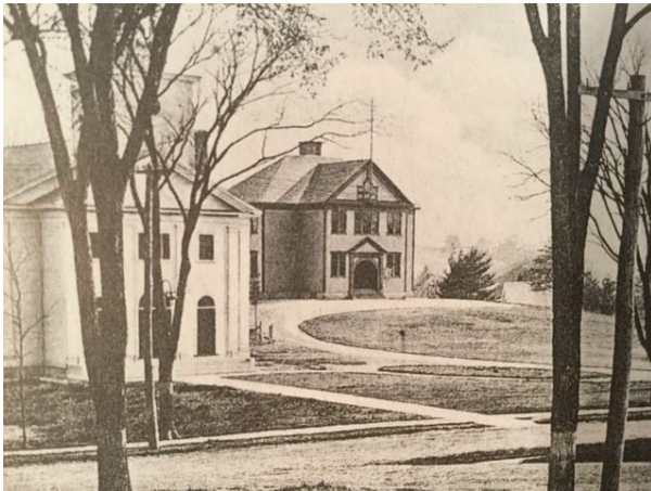
Image 1: Historic photos depict a distant flagpole mounted high in the entry pavilion.
