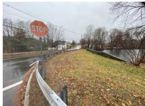
The guardrail along the Shaw Conservation Area presents a significant barrier to even informal pedestrian activity, and the large curb radius further exacerbates walkability issues.
