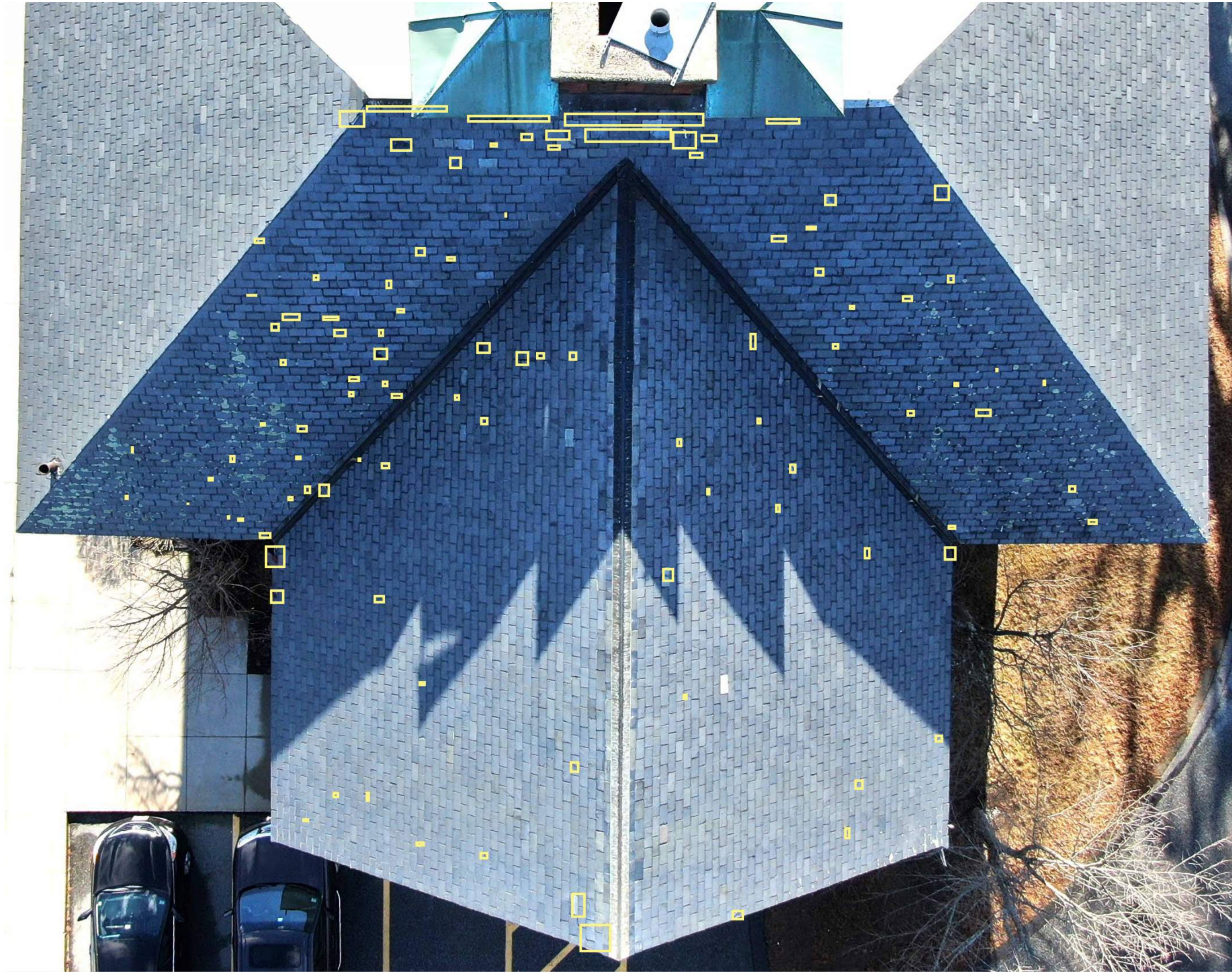
① North Roof Areas of Damage 1/8" = 1'-0"
