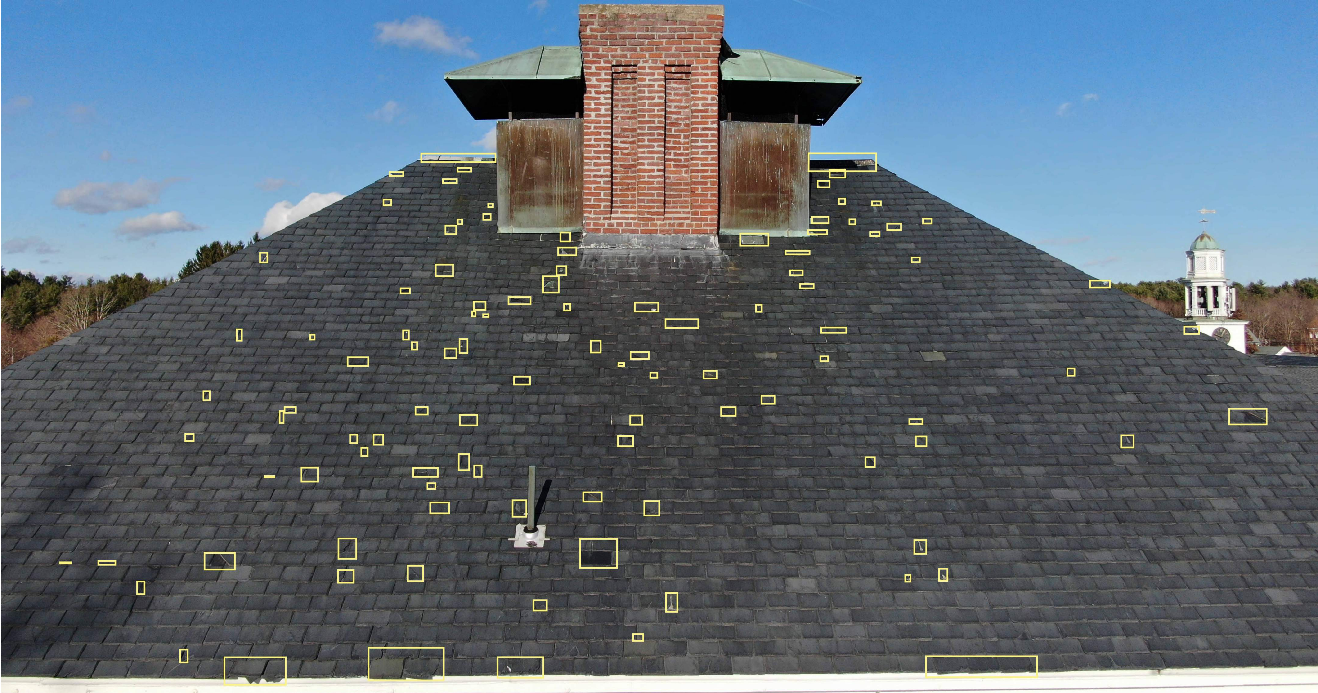
1 South Roof Areas of Damage 1/8" = 1'-0"
