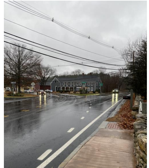
The new sidewalk ends abruptly before the Pleasant and Main Street intersection
