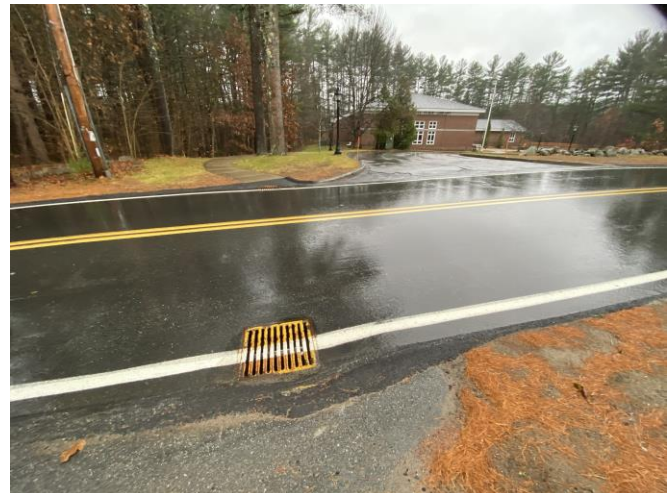
The crosswalk between Highland Street and the Dunstable Free Public Library was recently paved over and never repainted; nonetheless, an inadequate curb ramp directs pedestrians to cross over a drain, presenting significant accessibility issues.
