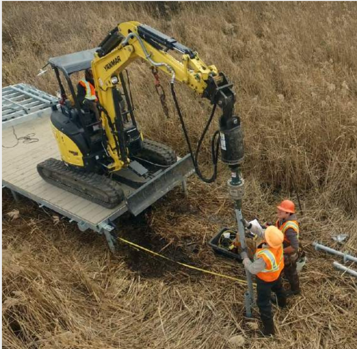
Modular "Top Down" Construction (Courtesy of Helical Drilling)
