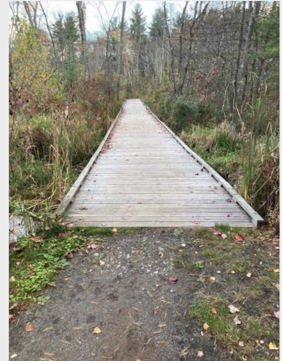
Pressure Treated Deck Southwest Park, Nashua, NH (2015 Construction)
