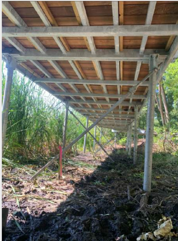
Modular Boardwalk Framing (Courtesy of Helical Drilling)
