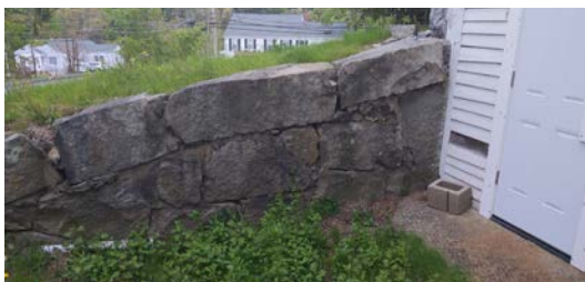
Image 4.04: A coarse stone retaining wall at the rear is in need of basic repointing.
