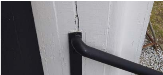
Image 2.08: Split wood jambs where the metal handrails are fastened should be monitored.
