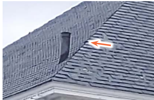
Image 1.01: Mitered slate hips have a visible joint that should be protected by interleaved flashings.
