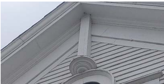
Image 2.07: A flagpole bracket and sleeve are the only evidence that one may have ever been present.
