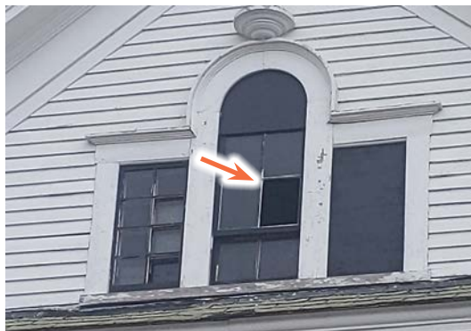
Image 3.02: The iconic Palladian window on the front facade requires complete restoration.
