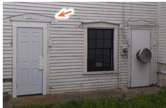
Image 3.06: Missing trim and an awkward selection of doors should all be replaced.
