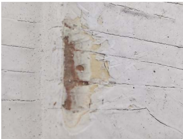
Image 2.05: The many layers of lead paint should be professionally analyzed to determine historic (and appropriate) colors.
