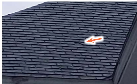
Image 1.03: Slates which are missing more than a quarter of their surface area should be replaced.
