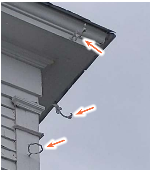
Image 1.07: Evidence of former half-round gutters and round corrugated downspouts are easily seen.
