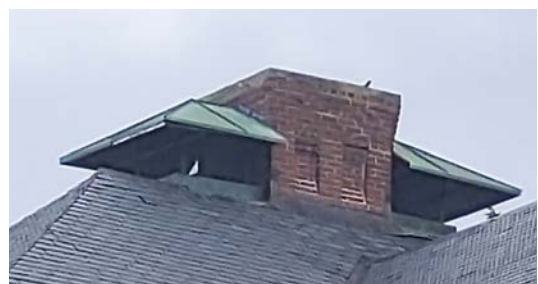
Image 1.04: The wide brick chimney exhibits partial repointing, but requires a full campaign.
