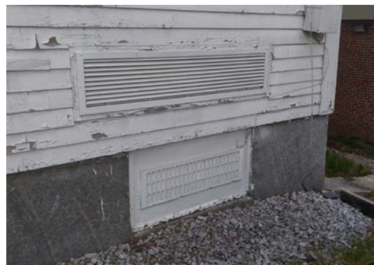
Image 3.07: Intake grilles at the building are part of the overall ventilation system, exhausting at the rooftop.
