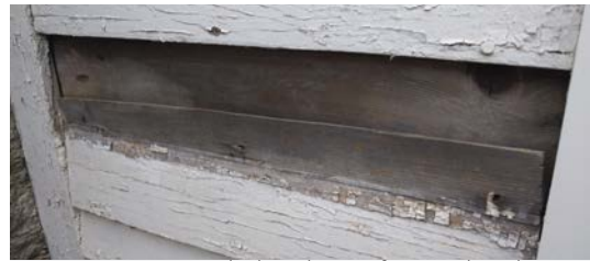
Image 2.02: Missing clapboards are infrequent but obvious, and should be replaced.
