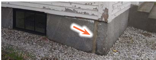
Image 4.02: Long, slender blocks of granite support the building's wood frame. Corners should be repointed.
