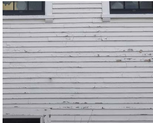
Image 2.01: The wood clapboards are well-maintained, but need a thorough repainting with historic colors.
