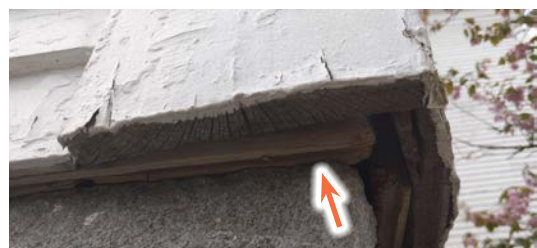
Image 2.04: Tongue-and-groove board sheathing is visible beneath the clapboards.
