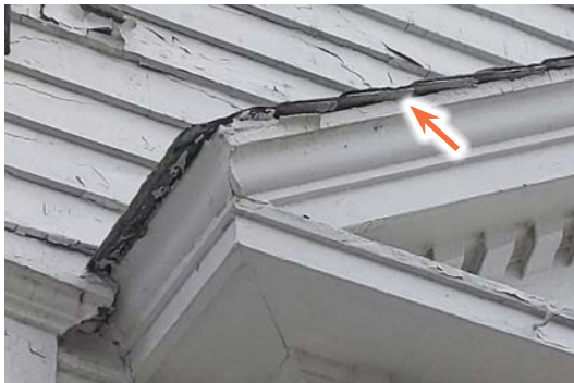
Image 1.05: A narrow band of slate shingles protecting the entry pediment peek out from over the crown moulding.
