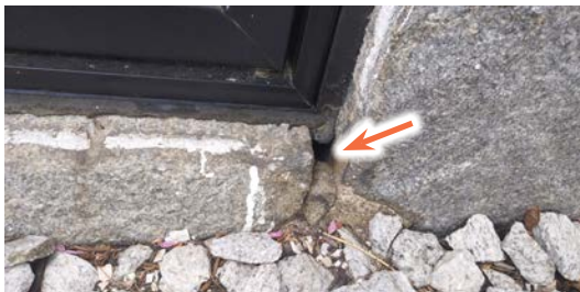
Image 4.03: Small openings in the basement window sill joints are a potential site for future leaks.
