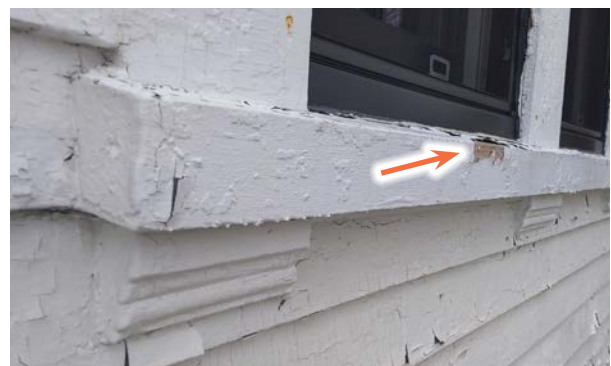
Image 3.04: Window trim details are generally well-maintained, but require thorough scraping and repainting.
