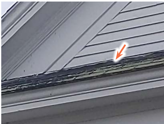
Image 1.06: Asphalt shingles at the horizontal cornice above the entry are delaminating and severely worn
