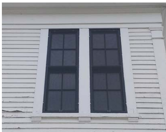
Image 3.03: Jet-black, modern aluminum clad wood windows are in excellent condition.
