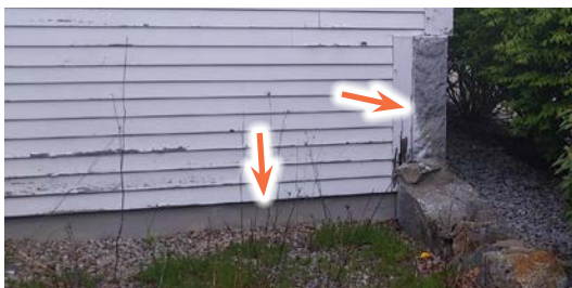
Image 4.01: A modern concrete foundation appears to have been installed with the new connector addition.
