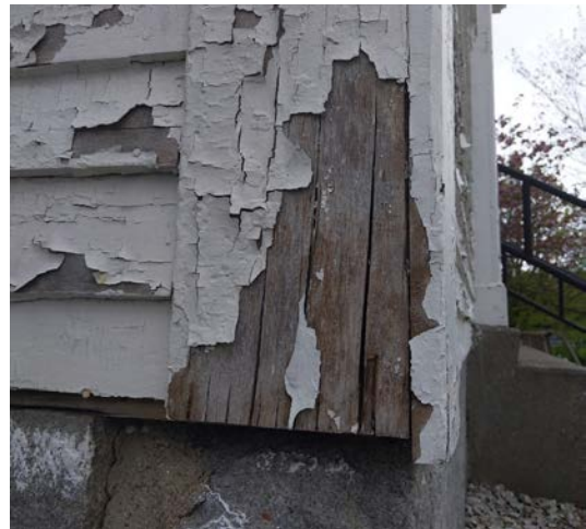
Image 2.10: Deteriorated cornerboards and skirts may require repair or selective replacement before repainting.
