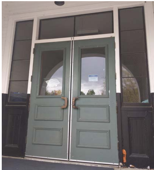
Image 3.01: Sage-green doors are protected by the alcove, but need a new coat of (appropriately colored) paint.
