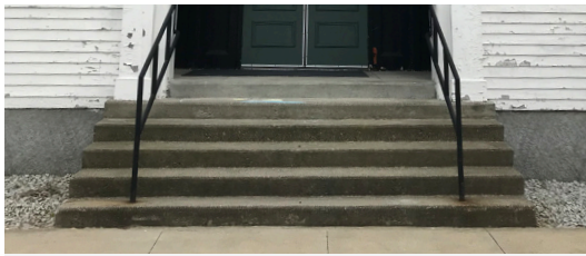
Image 4.01: The concrete steps are unmarred and intact, however dull they may appear.
