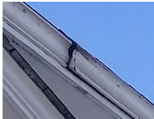
Image 2.11: Loose or missing trim should be refastened after making any repairs.
