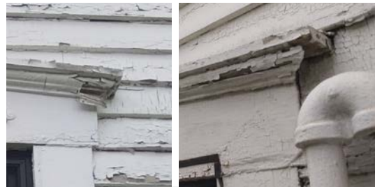
Image 3.05: Deteriorated window trim is typically limited to the crown mouldings.
