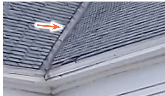
Image 1.02: The open slate valleys are flashed by a strip of flashing with a pronounced 'V' to stop splashing rain.
