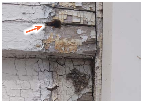
Image 2.03: Ferrous nails have a tendency to rust and split open clapboard when exposed to moisture and air.
